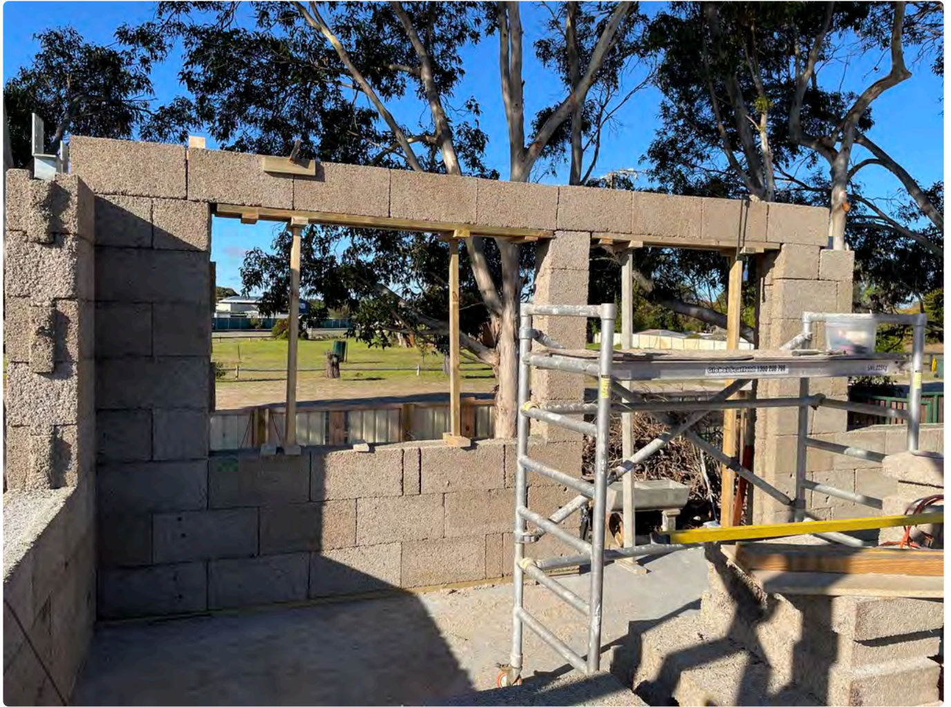
Timber lintel block supports.
