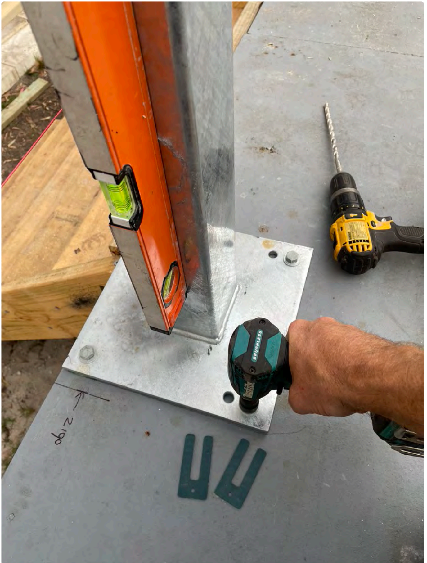
(the screws are connected to joists that are positioned under the floor)
